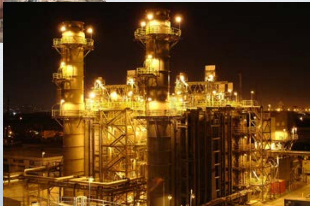
City of Vernon Light and Power Malburg Generating Station Vernon
