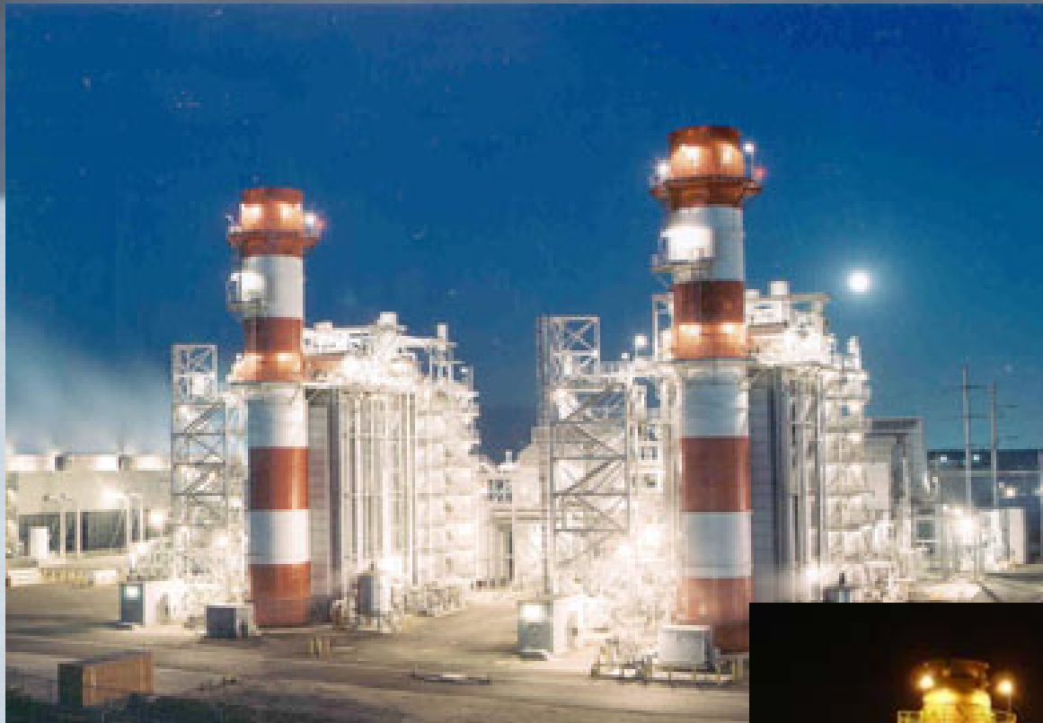
LADWP Valley Generating Station Sun Valley
